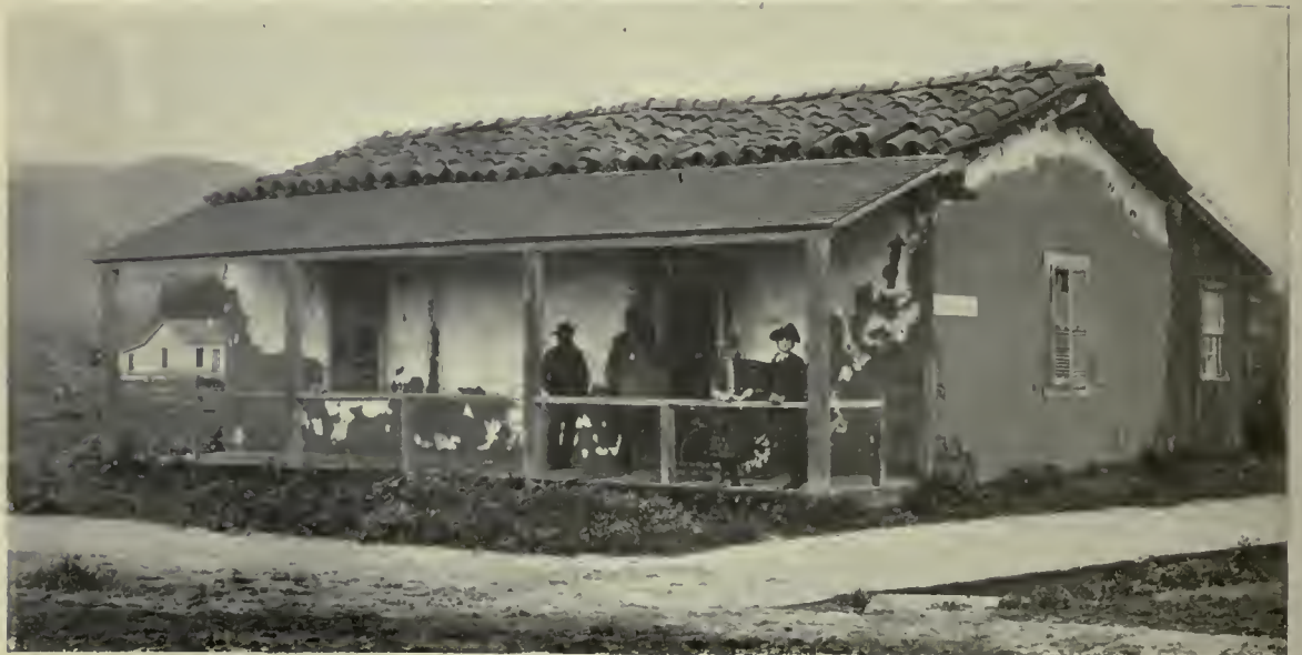
LAST ADOBE HOUSE IN VENTURA
